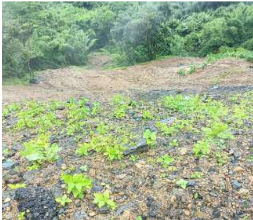
2. Pic: Spoil Bank No. 06, Ambyu Village Area, Siaha District
