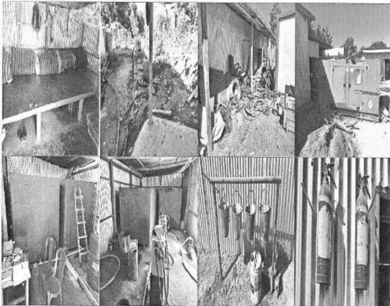
(1-2) Operator Camp residing/ washing area, (3) Poor housekeeping at store, (4) To increase DG stack height, (5-8) Fuel storage tank, Empty fire bucket & unspecified fire extinguisher
