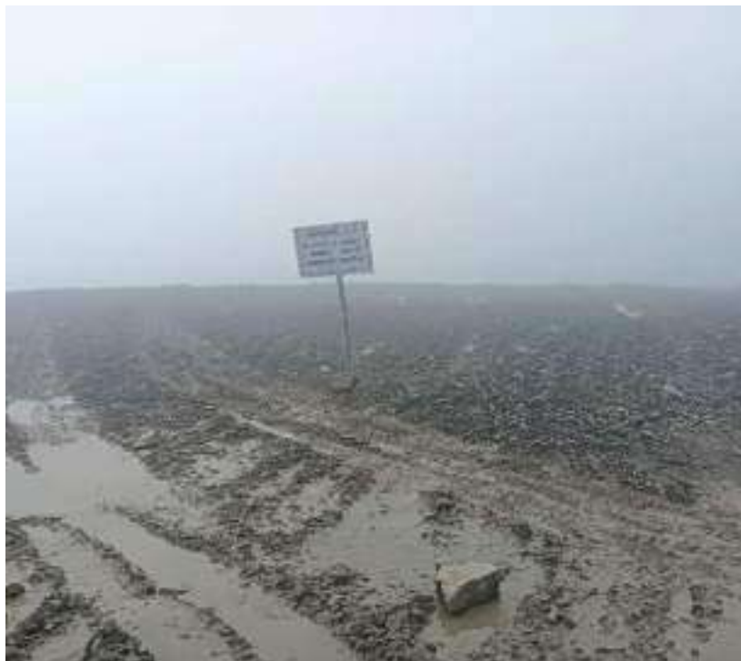
1. Pic: Spoil Bank A-2, Chawnhu Village area, Lawngtlai District
